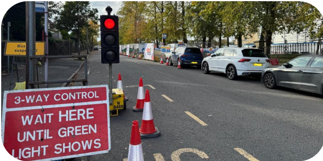
A photo of temporary traffic lights on Godfrey Road
