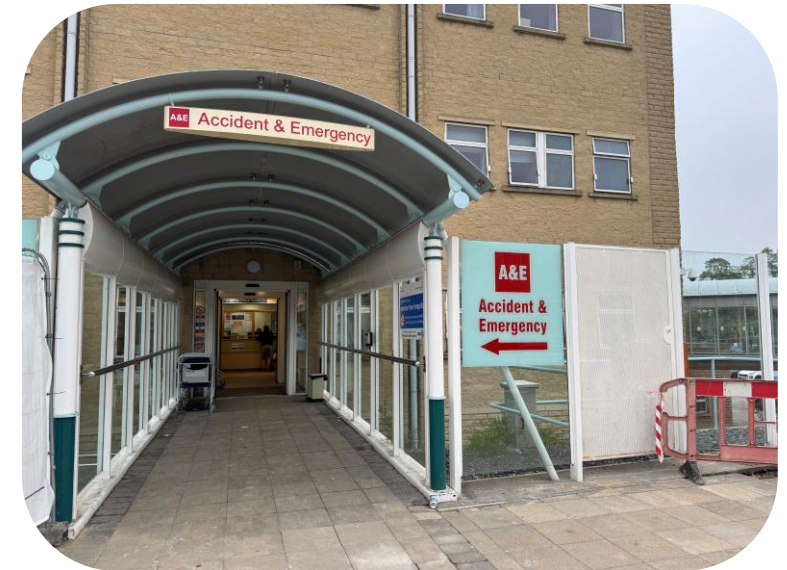
A photo of the A&E entrance at CRH with the canopy now removed
