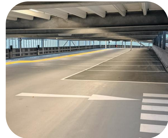
Images: (top) the outside of the car park and stairwell, (bottom) one of the floors in the car park
