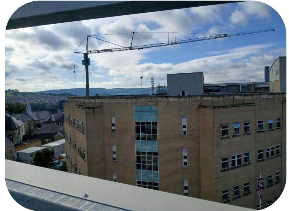
The crane at CRH lifting steel above the roofline as part of the internal development works
