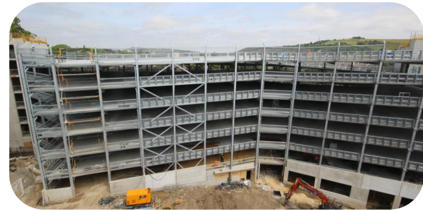
Photos: top – one of the completed concrete floors in the car park, and bottom – a photo taken from the time-lapse camera in mid-June 2026.
